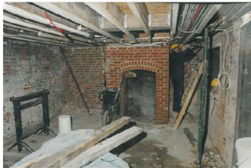
Undated record photo (assumed 1990) at ground floor, north wall, showing work to first floor joists
