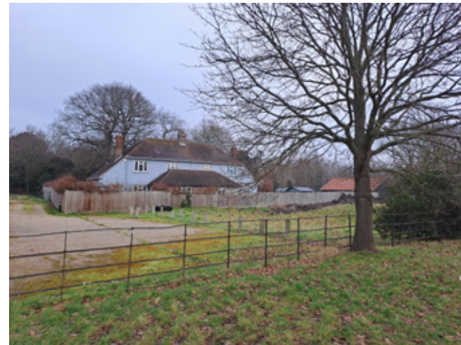
Figure 93 The setting of The Temple to the rear, with the Keepers' Lodges.
