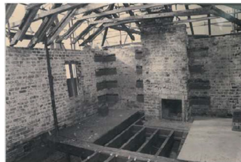
Record photo from 1990. First floor, north and west walls showing elbow ties
