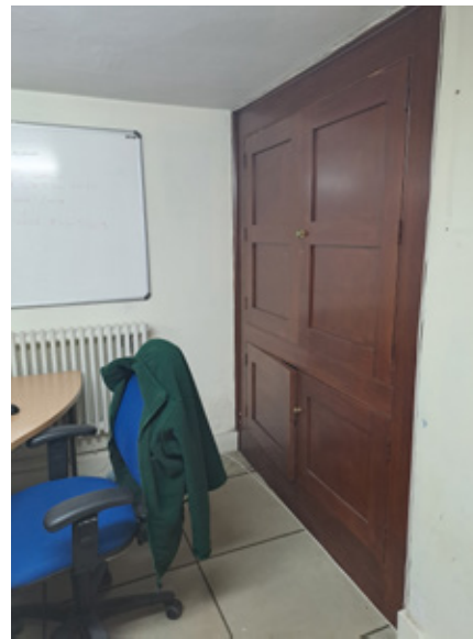
Figure 29 Modern joinery spanning a previous opening into the single-storey extension to the north, removed in the 1950s.
