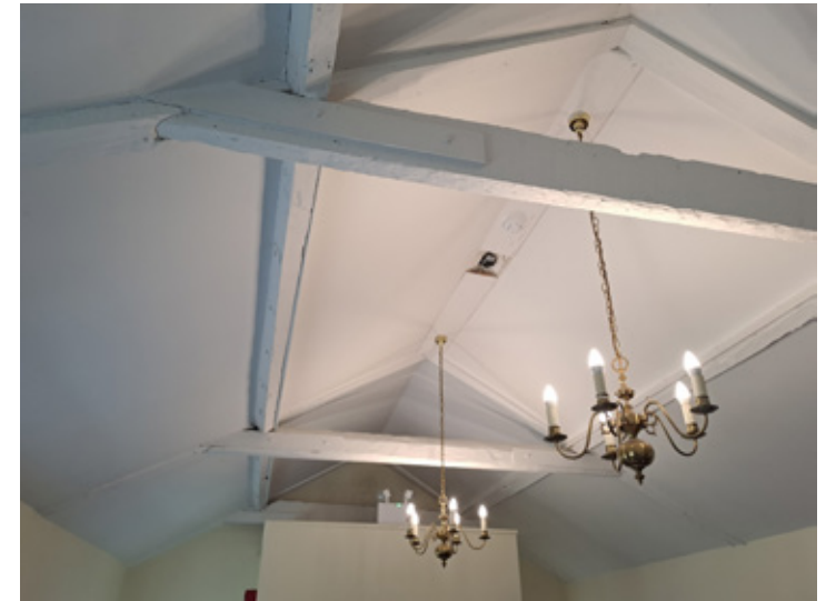
Figure 14 Rafters in the northern wing, upper-ground floor.
