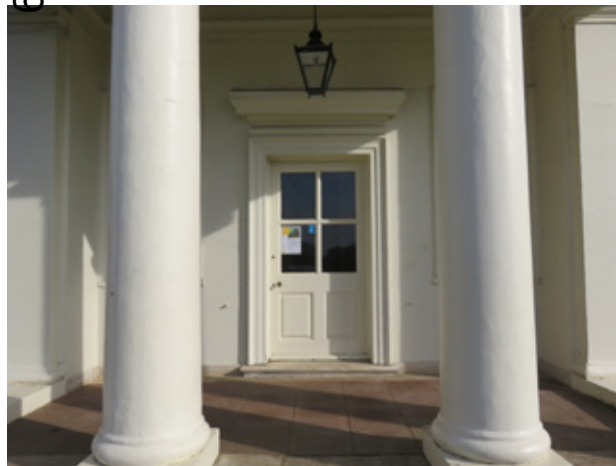
Figure 06 The main entrance door to upper-ground floor level
