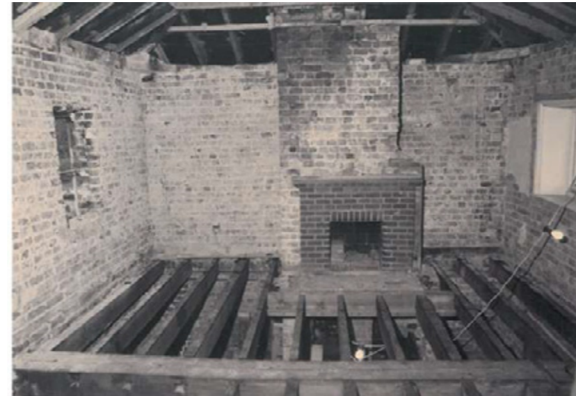
Record photo from 1990. First floor north wall
