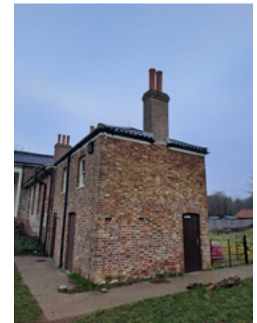
Figure 09 The south elevation of The Temple, showing the modern door providing entry to the men's public toilets at lower-ground floor level
