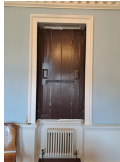
Figure 12 Wooden folding shutter in the east elevation on the upper-ground floor.
