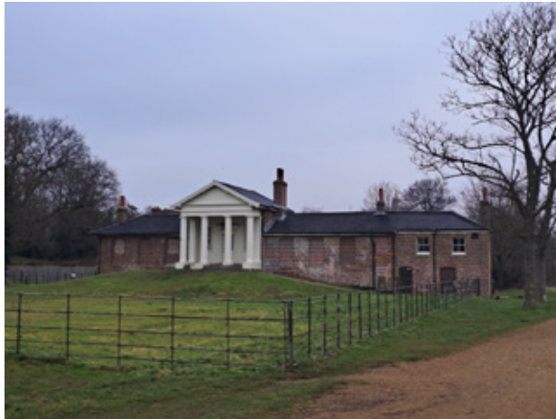
Figure 03 West elevation of The Temple
