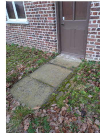
Figure 08 Paving laid to improve access to The Temple in the late 1990s
